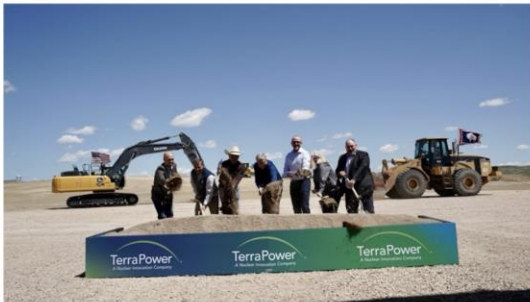
The groundbreaking ceremony marks the start of non-nuclear construction work at the site (Image: TerraPower)
