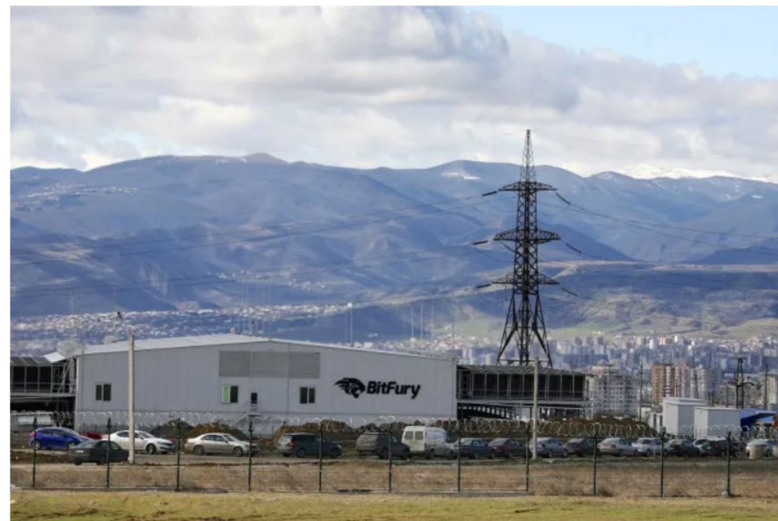
Bitfury's facility in the outskirts of Tbilisi. Source: Andrew North for NPR.
