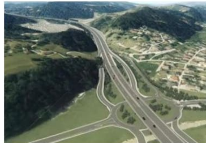
Construction of Highway through Velenje
