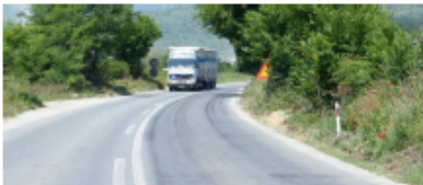
Insufficient stopping site distance in curve
