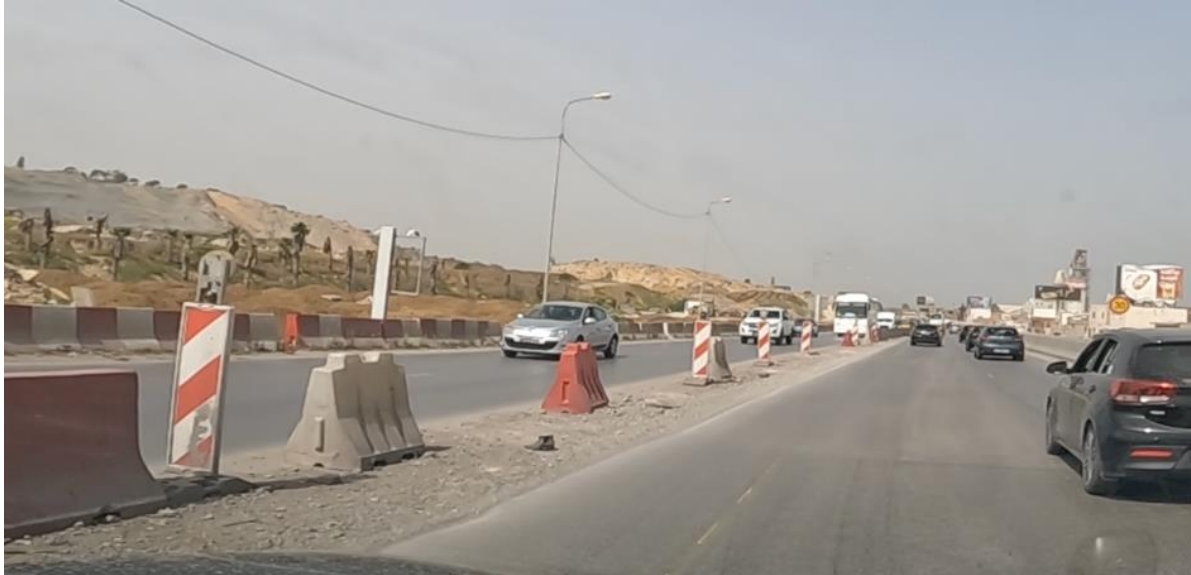
Unsafe median separators
