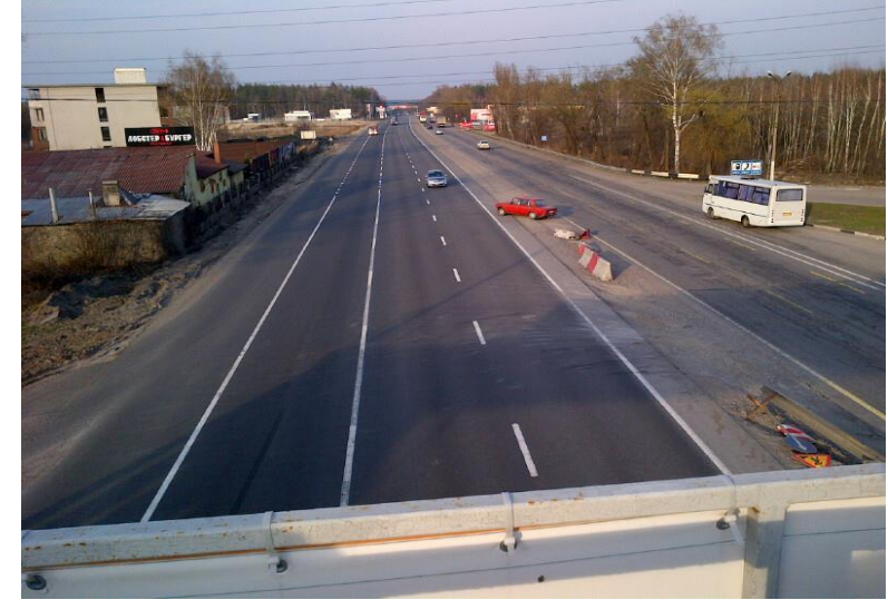
Inadequate provisions for left turns
