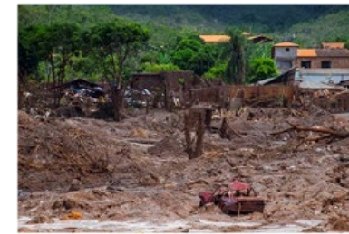
Brumandinho dam collapse (Brazil, 2019)
