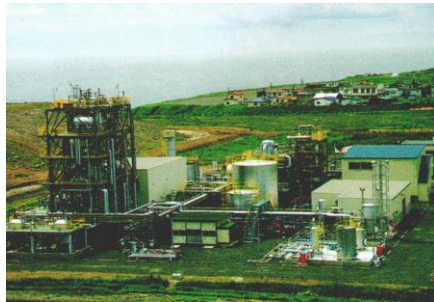
Methanol Production Plant
