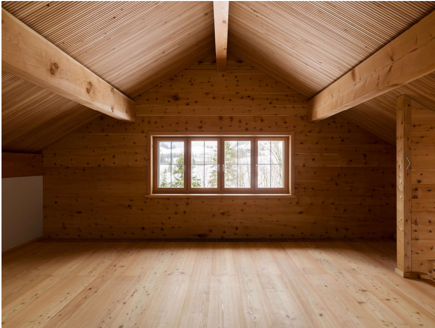
Fig. 17 Attic floor in solid Douglas fir and larch.
