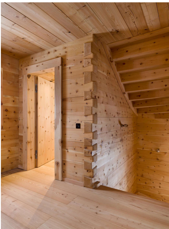
Fig. 15 Steps and door to the wet room on the first floor
