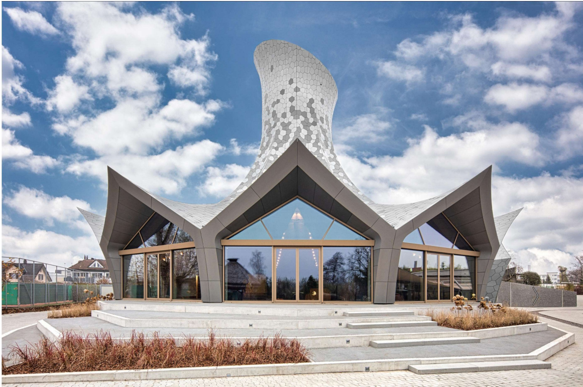
Fig. 8 The building's design picks up on the traditional circus theme of the magician's hat.
