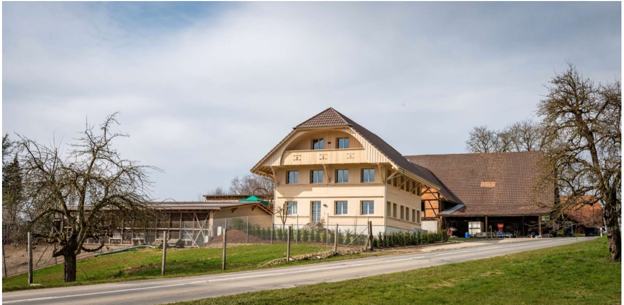
Fig. 22 The new building complements the existing barn and stables.
