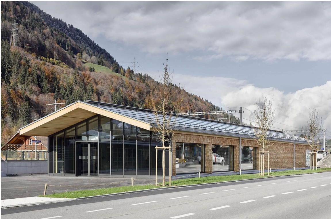
Fig. 30 The cladding of the façade with roof shingles provides a connection with traditional woodwork in the region.
