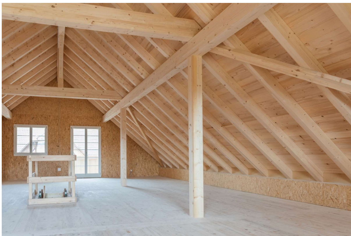
Fig. 25 The generously sized attic floor with the solid-wood roof truss.
