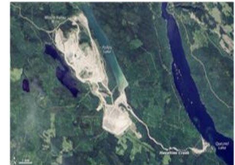
Mount Polley tailings dam break (Canada, 2014)
