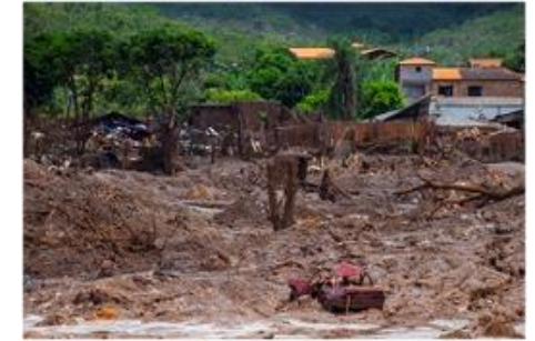
Brumandinho dam collapse (Brazil, 2019)
