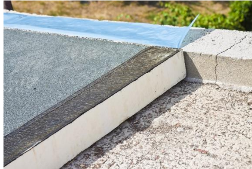
Figure 15. Flat roof - insulation of the exterior surface 23
