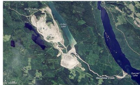
Mount Polley tailings dam break (Canada, 2014)
