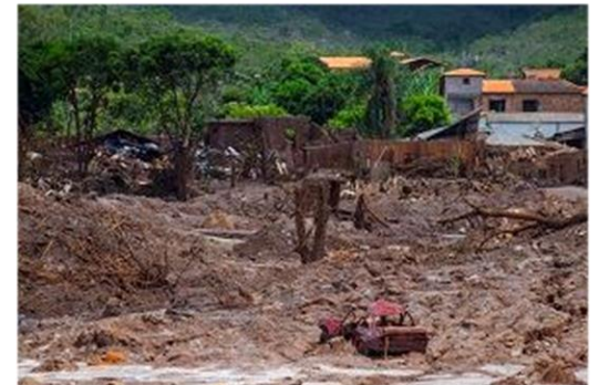
Brumandinho dam collapse (Brazil, 2019)
