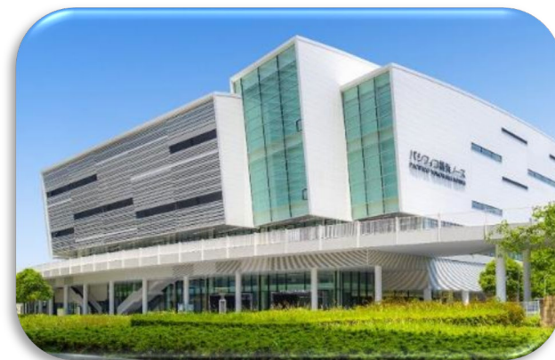
Pacifico Yokohama North
