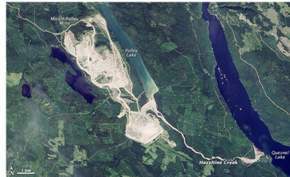
Mount Polley tailings dam break (Canada, 2014)
