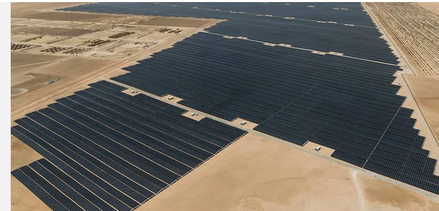
1.17GW Nour Abu Dhabi Solar PV plant
