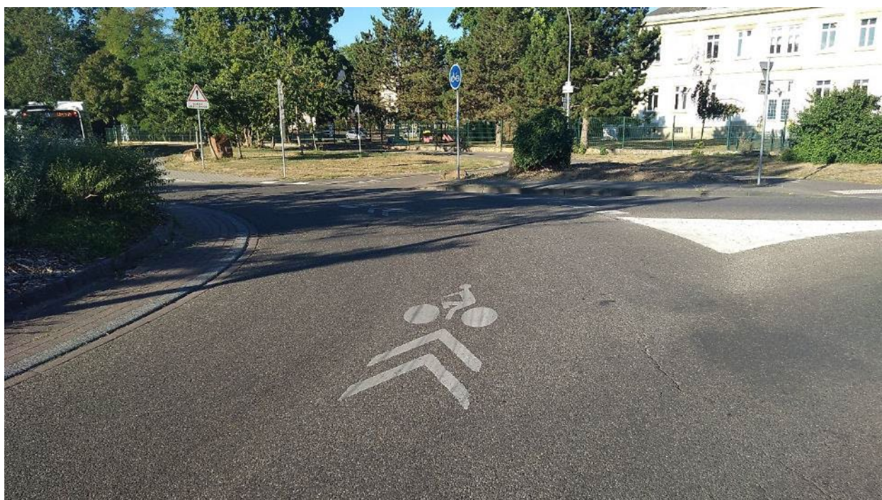
Figure 3. Sharrows on a roundabout advise cyclists to ride in the middle of the lane. Strasbourg, France. Source: Aleksander Buczyński
