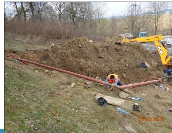
Figure 12. Gas pipelines affected by landslides – area I PhD. Thesis: K. Alexandra, 2018
