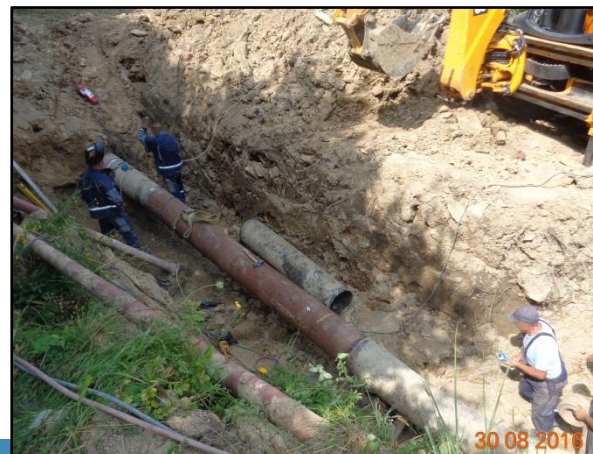
Figure 12. Gas pipelines affected by landslides – area I PhD. Thesis: K. Alexandra, 2018
