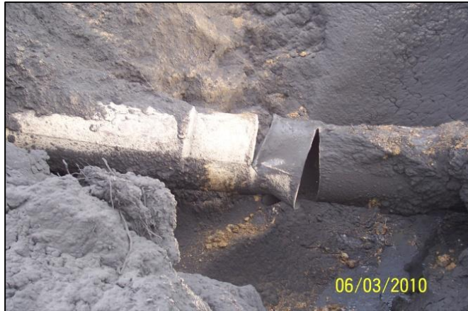
Figure 14. Gas pipelines affected by landslides – area 3
