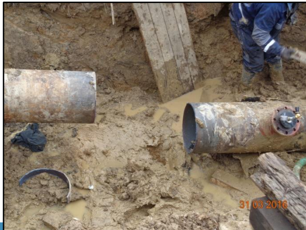
Figure 12. Gas pipelines affected by landslides – area I PhD. Thesis: K. Alexandra, 2018
