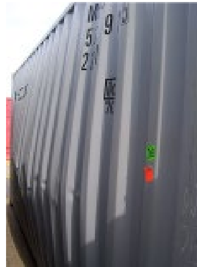
Figure 7.53 - Damaged side wall following road transport
