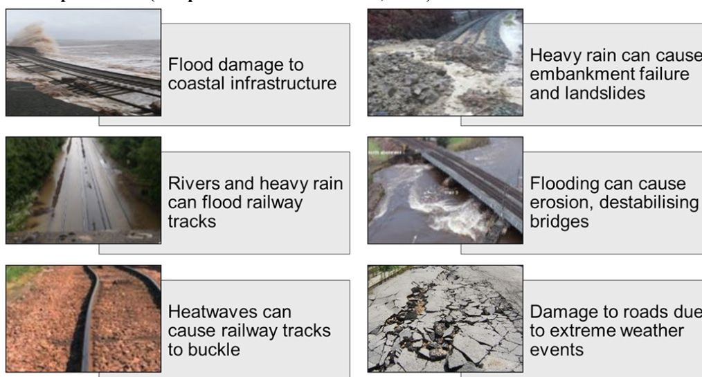
Some key examples of the impacts of weather and longer-term climatic change on different transport assets (Adapted from Ferranti et al., 2021)
