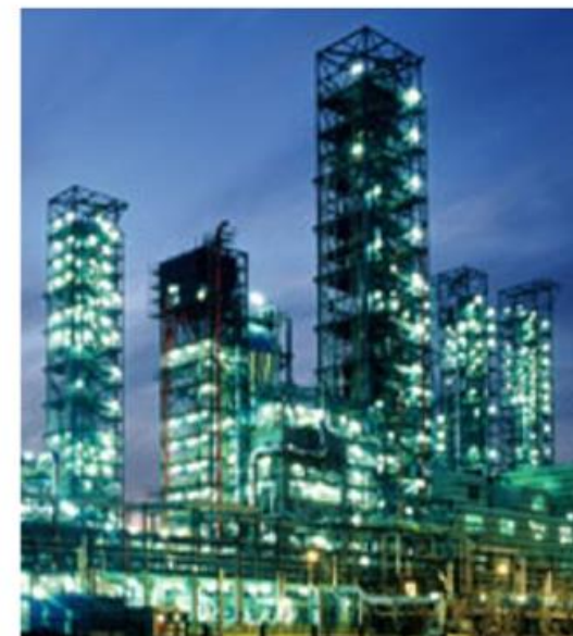
Sinopec Refinery, China
