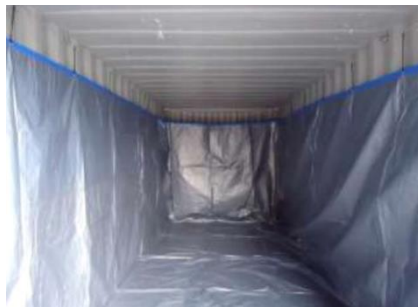
Figure 42 Liner in place
