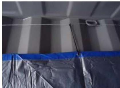
Figure 43 Supporting the liner
