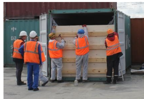
Figure 46 Rear false bulkhead
