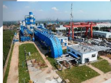
GaoHe mine, 2014 1,020,000 Nm 3 /h 20 MW steam turbine
