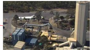
West Cliff mine, 2006 250,000 Nm 3 /h 6 MW steam turbine
