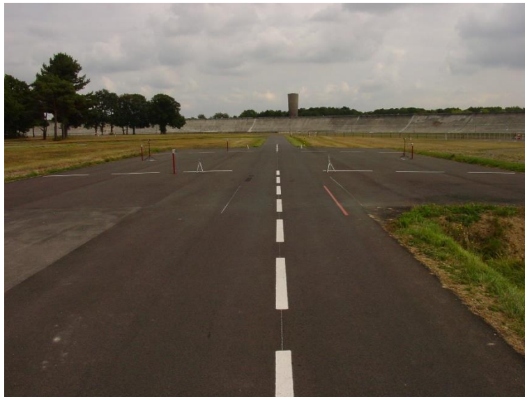
Figure 2.2-3 : UTAC sound track for Rolling Sound test
