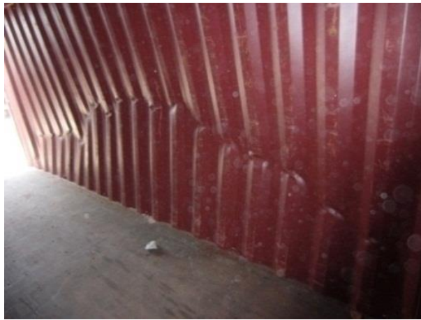
Figure 7.50 Damaged CTU side wall
