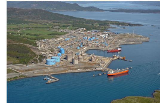
Picture of the gas and condensate processing plant at Kårstø (Photo: Øyvind Sætre - Gassco)
