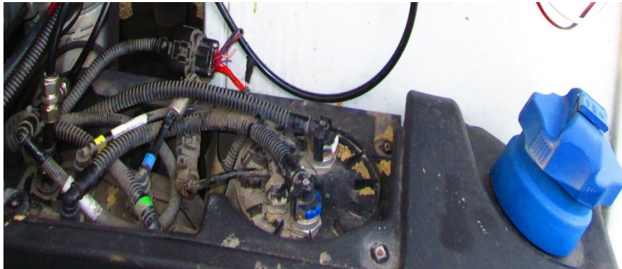
Figure 23 Visual inspection: Urea Fuel Tank
