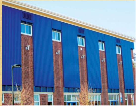
New Hingham Elementary School in Hingham, Massachusetts
