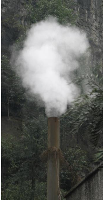
Coal mine methane from a vent stack, Source: Global Methane Initiative.
