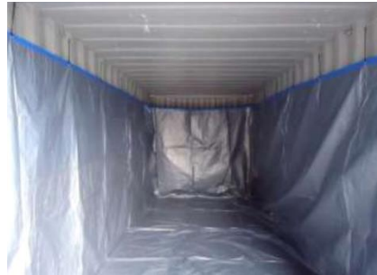
Figure 42 Liner in place
