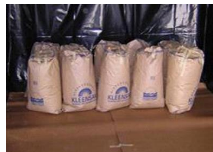
Figure 44 Bagged sawdust prior to laying
