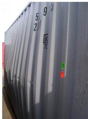
Figure 7.53 Bulging wall
