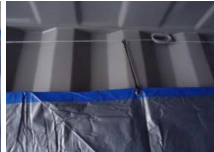
Figure 43 Supporting the liner
