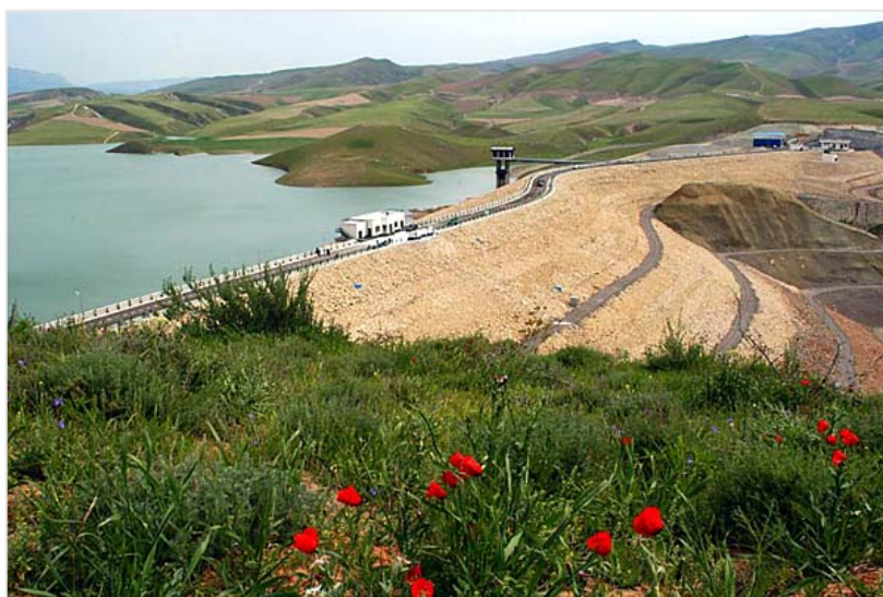
Joint Iran-Turkmenistan reservoir dam on the TEJEN River/GERIRUD
