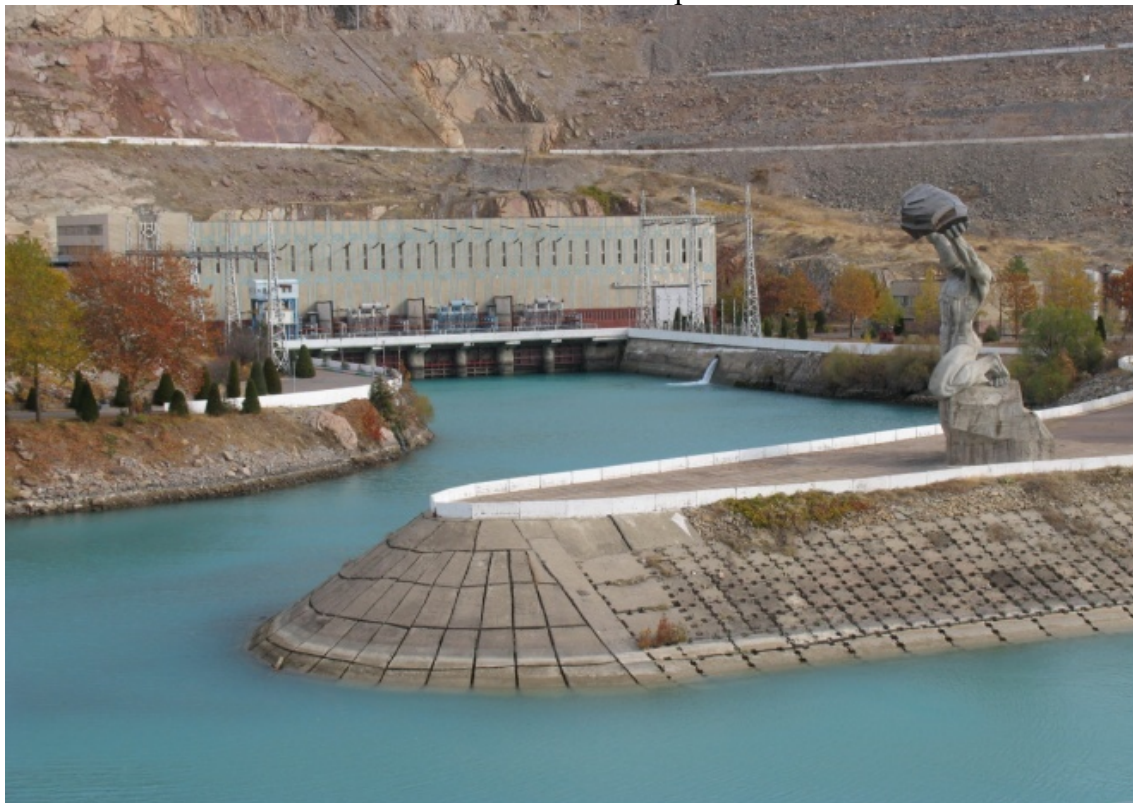
Charvak hydroelectric power plant on the CHIRCHIK river, Uzbekistan (Dam height-168 m; volume of water-2006 million.m 3 )
