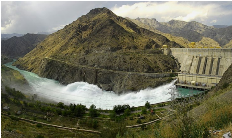
KURPSAY hydroelectric power station on the NARYN River, KYRGYZSTAN
