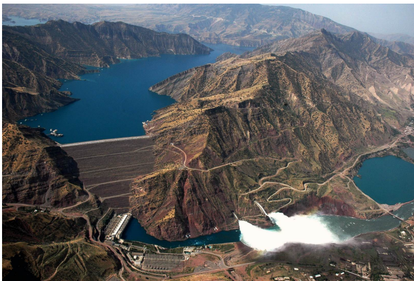
NUREK hydroelectric power station on the VAKHSH river, TAJIKISTAN
