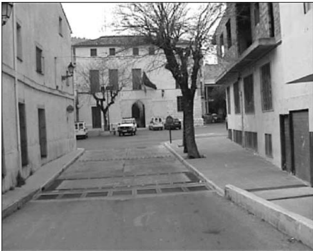
Figure 12 A view of Sumacárcel main square from its access across the bridge.
