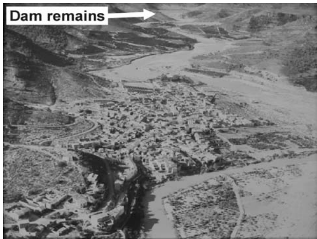
Figure 4 The town of Sumacárcel after the flood, looking upstream.
