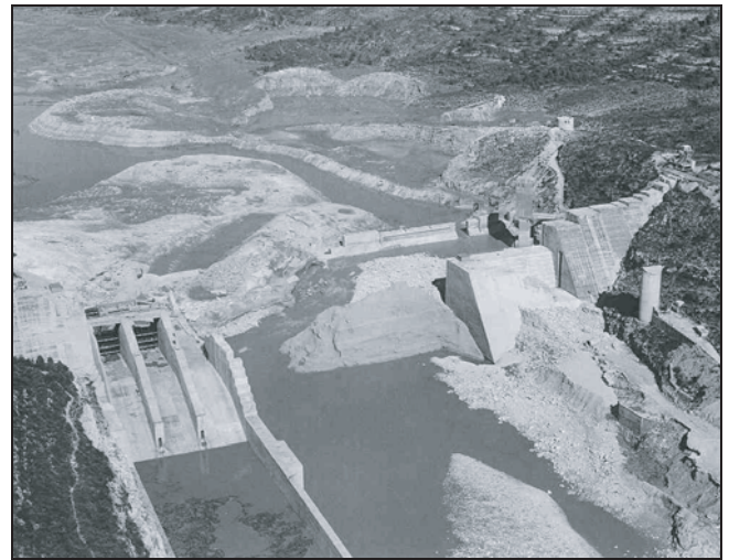
Figure 1 The remains of Tous Dam after the failure looking upstream (from Estrela, 1999).
