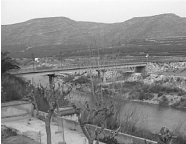
Figure 11 Present day view of Gauge 1 location (riverbed at the bridge) looking upstream.
