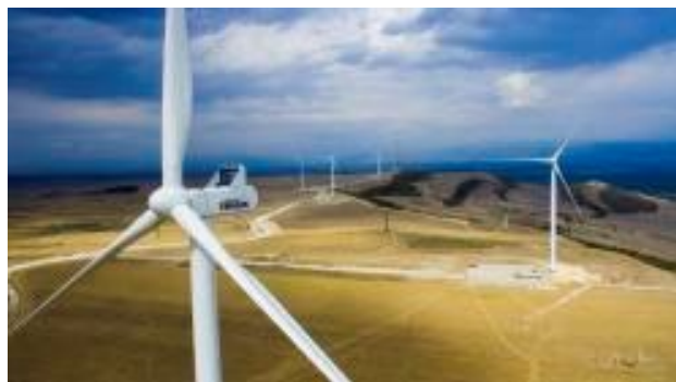
Kartli Wind Power Plant
