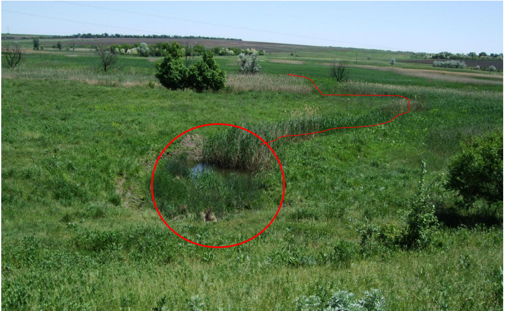
Filtration of water through a dam and outlet in the form of a spring. (View from the dam)
