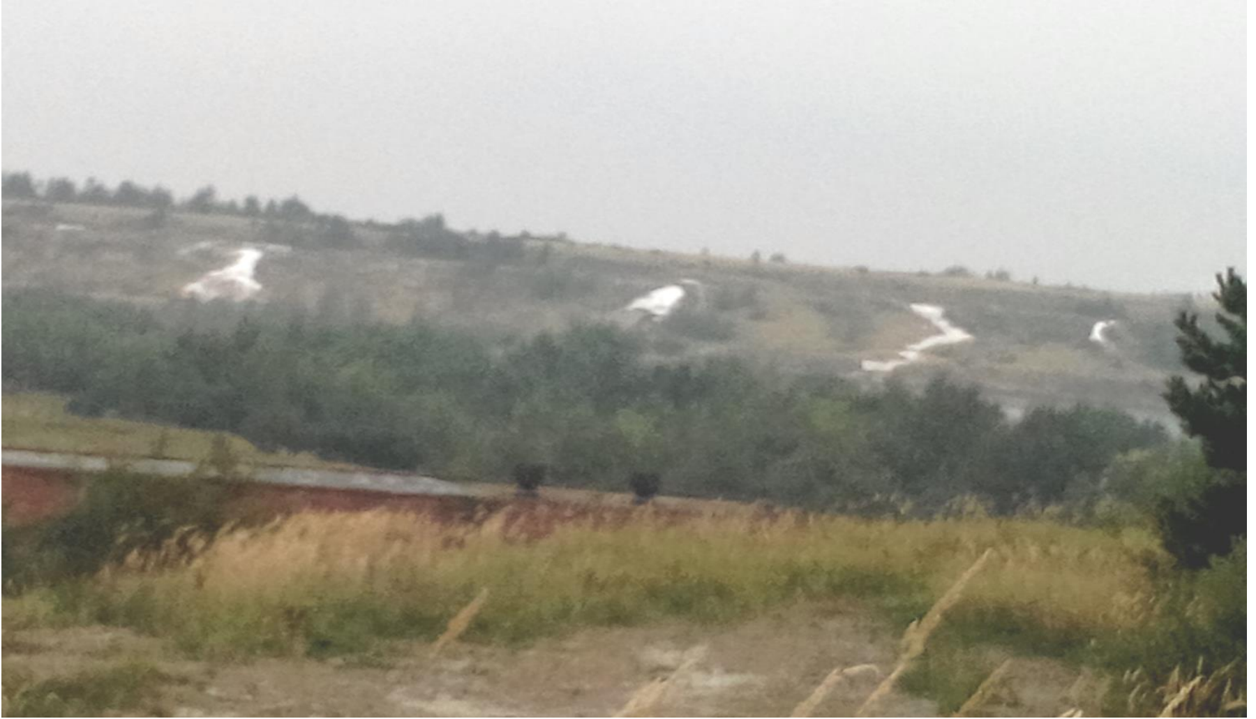
The outer slopes of the tailings dam.
