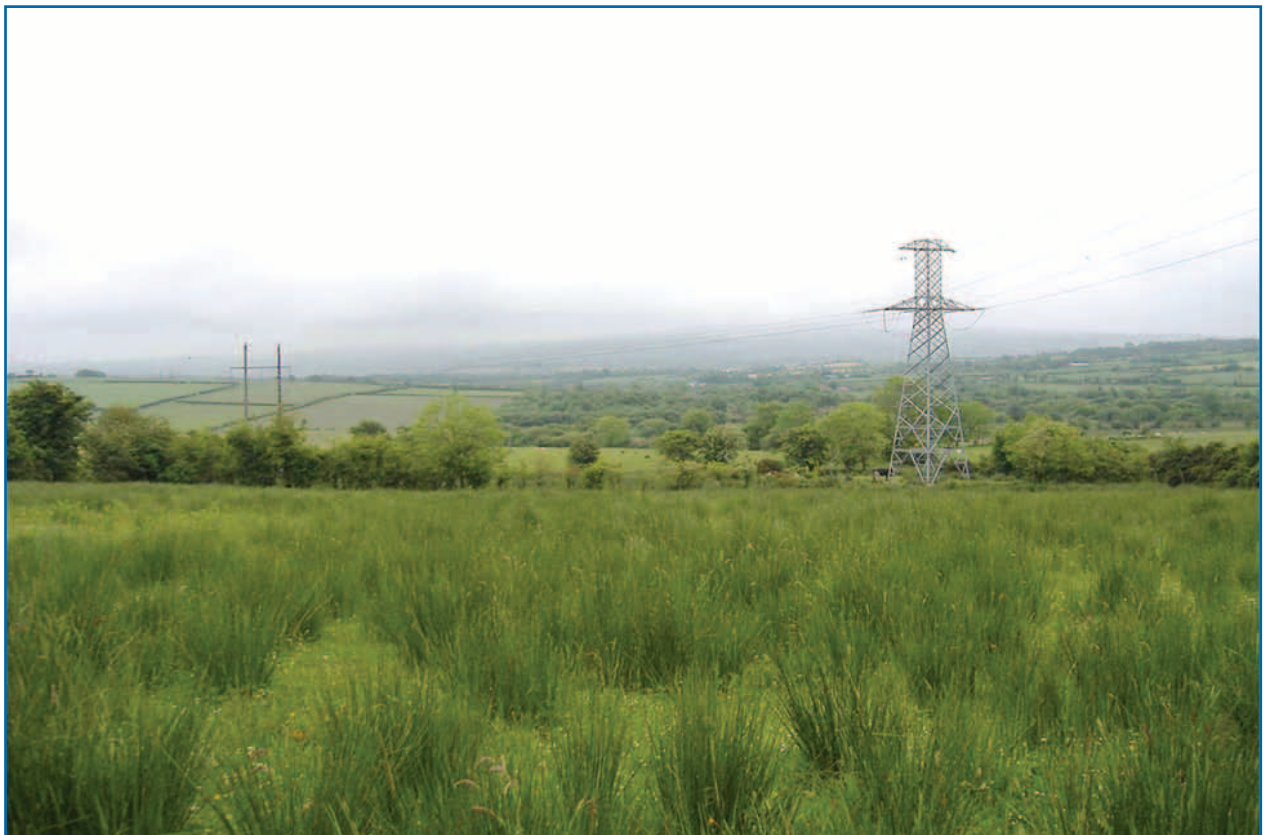
Figure 8.4 110 kV line lattice steel angle tower
