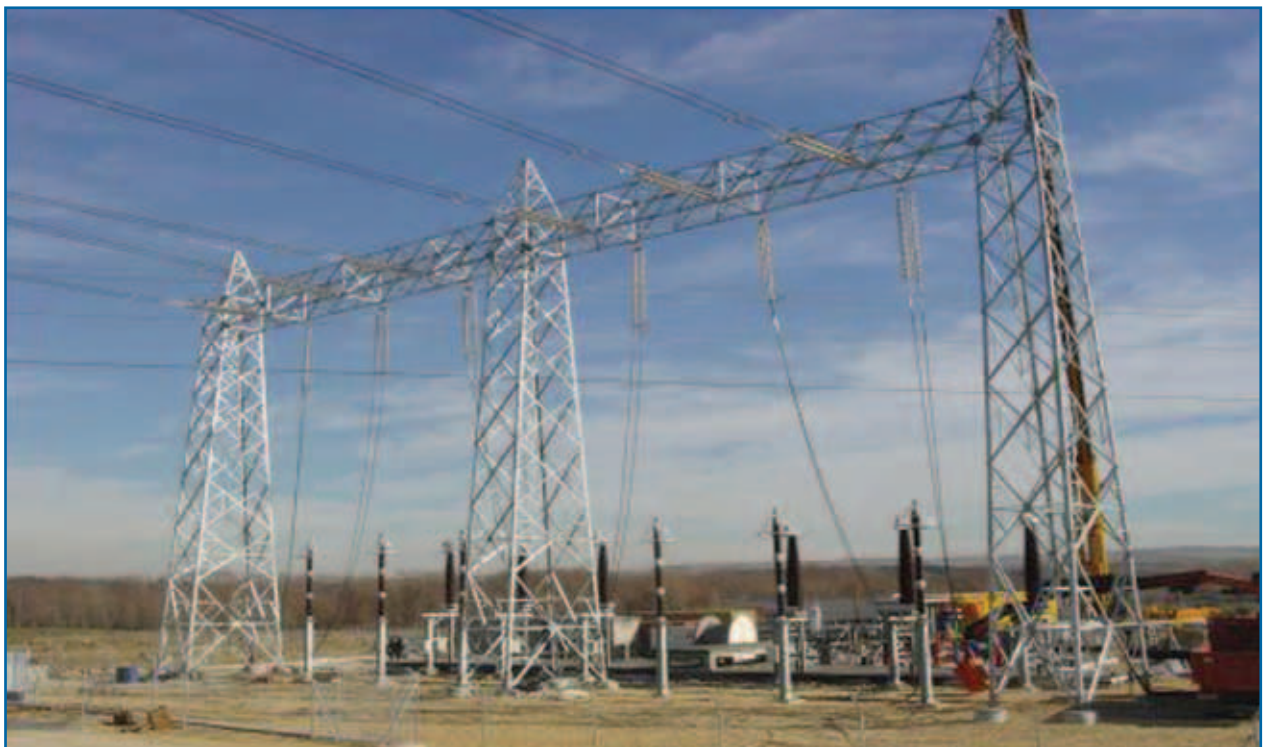
Figure 8.1 Typical Line/Cable Interface Compound
