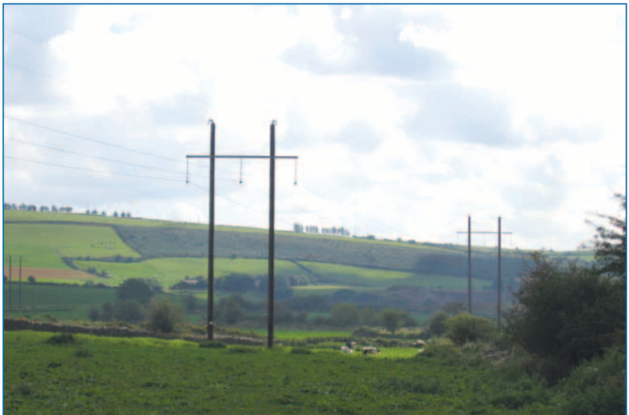
Figure 1.3: Single Circuit 110 kV Overhead Line Design
