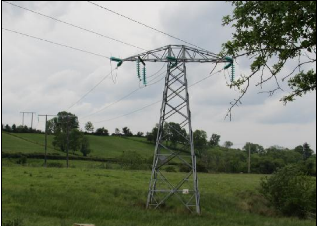
Figure 8.9: Photograph of a 110 kV Non-Earthwire Angle Mast
