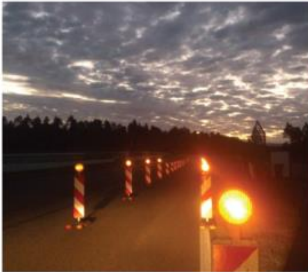
Figure 9: The built up construction zone at the Hockenheimring.
