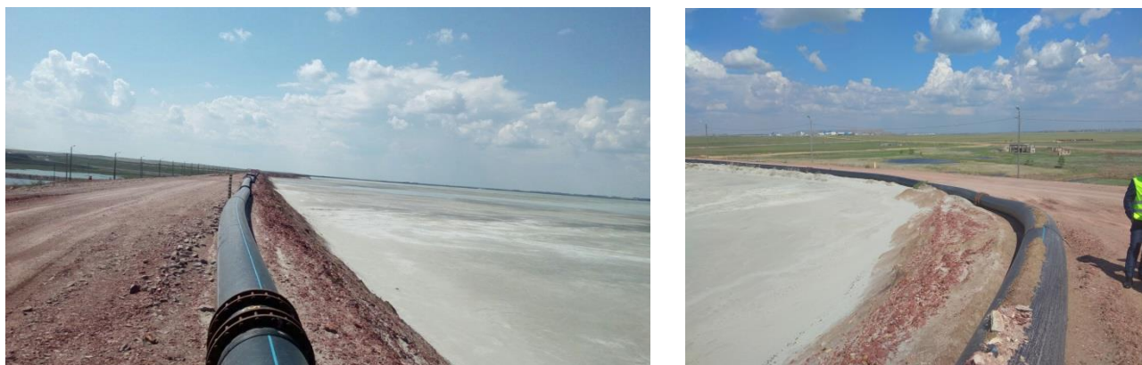
Figure 2: Views to the flotation TMF from the point 1 (see Fig. 1,b) to the west (a) and north-east (b)
