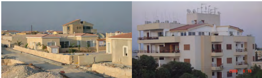
(left); good quality villas constructed without a building permit (right) 28
