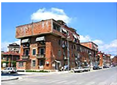
FIGURE 3: Additional unauthorized top of an existing building 14
