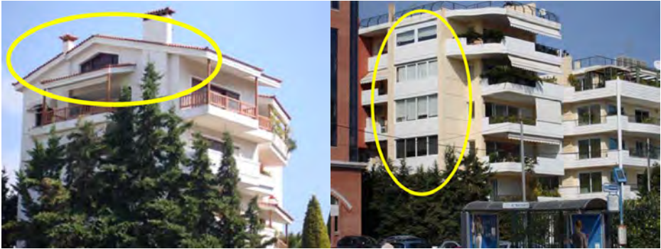
FIGURE 17: Illegal room under the roof of the building (left); Enclosure of semi-open areas that are within the ratified outline of the volume of the building (right) 46
