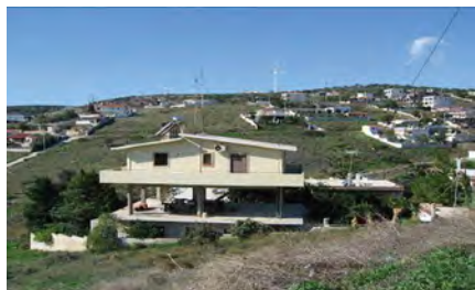
FIGURE 13: Informal buildings in unplanned areas without a permit (photo by C. Potsiou)
