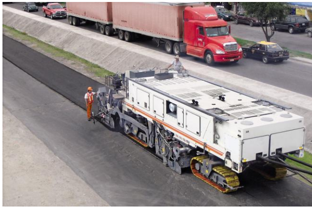
Cold recycler in operation
