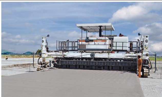
Slipform paver in operation
