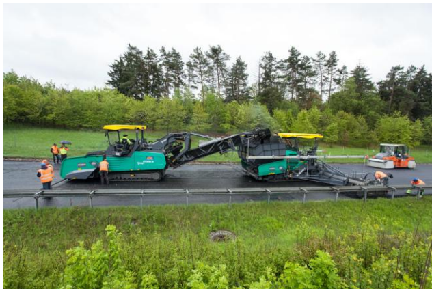
Feeder, asphalt paver and pneumatic-tyred roller in operation
