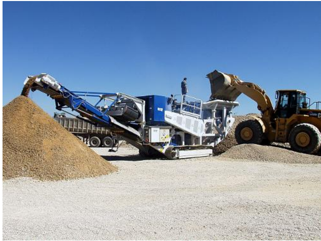
Mobile crusher in operation
