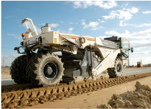
Cold recycler / soil stabilizer in operation
