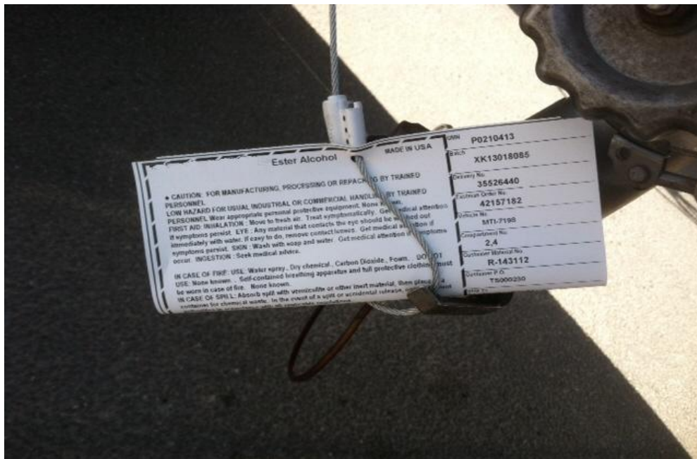
Figure 2. GHS information provided on a tag at the loading/unloading location
