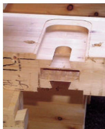
FIGURE 4.3.1 Notched joints typical of post & beam construction in Japan
