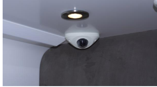
Figure 6.2 The CCTV camera monitors and records activity remotely. Alerts are sent on motion activation.
