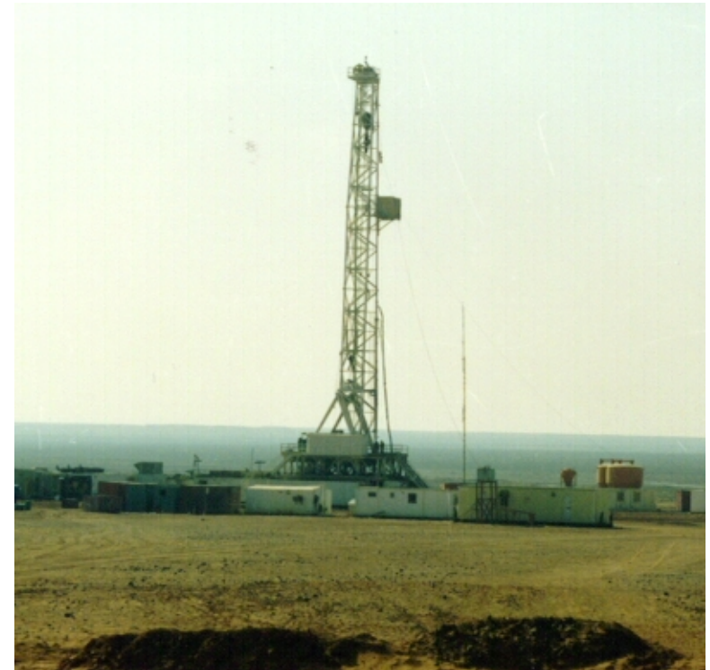
Exploration water drilling to 1500m depth
