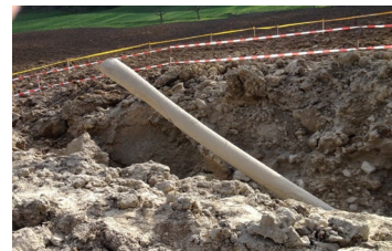
2'400 km gas and oil pipelines
