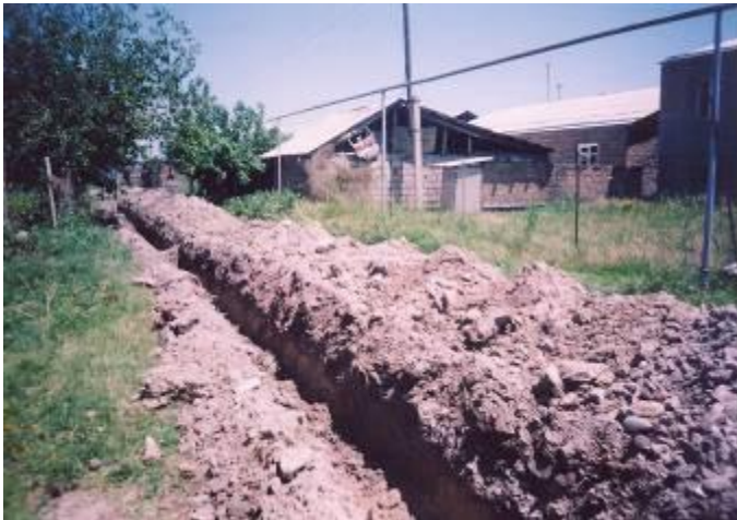
Providing drinking water supply system
