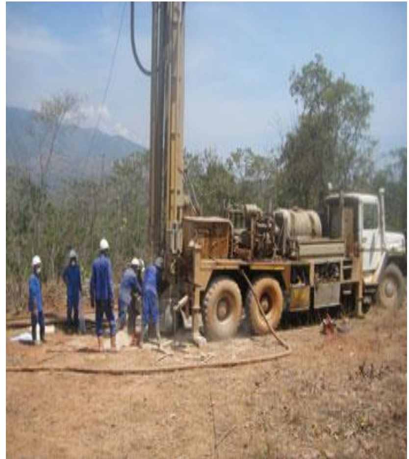
Works in Progress at Livingstonia Site
