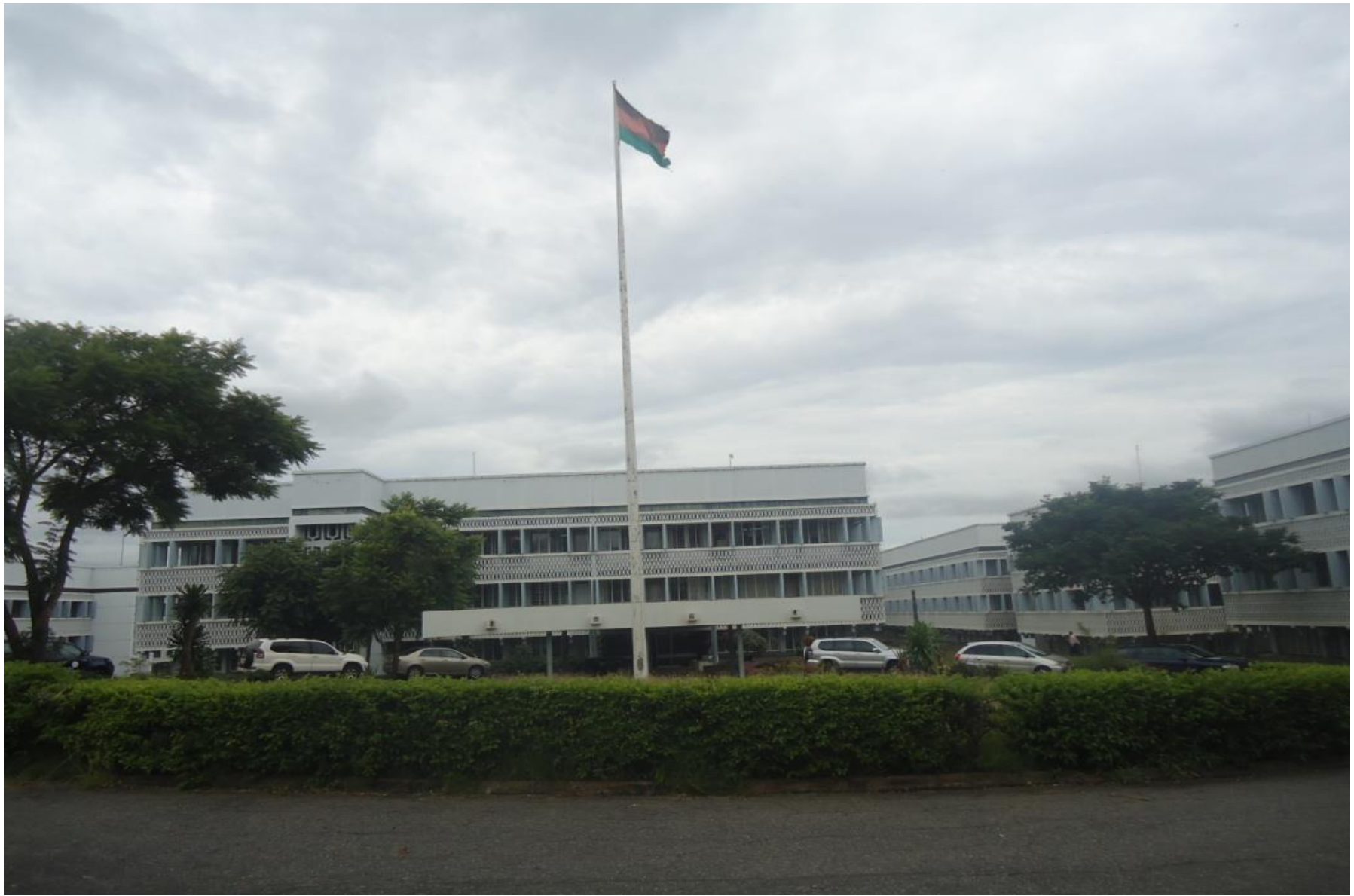
Ministry of Mining Headquarters, Lilongwe, Malawi
