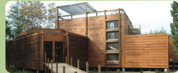
Administrative and Visitors' buildings of Kolkheti National Park - Wood service
