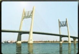
Highway Western High-Speed Diameter
