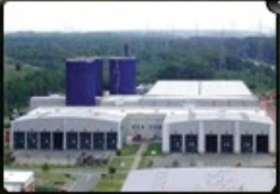
Waste processing plant in Yanino
