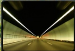
Orlovsky Toll Tunnel under Neva River
