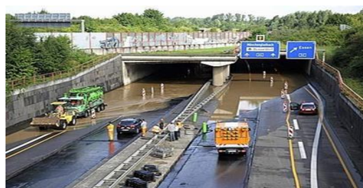
Inundation of tunnels
