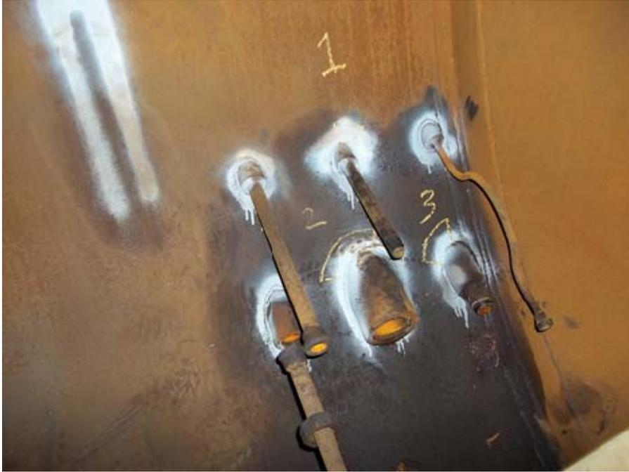
Following the initial indications of cracking light grinding of the surface was undertaken to ensure that it was not just weld overlap, however it was confirmed that all three were hairline cracks (the white background paint and black indicator has now made these very visible to the naked eye).
