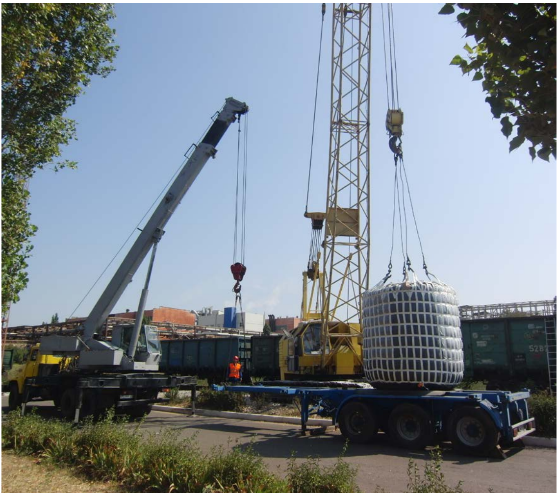
Photo 1 A general view of testing complex
